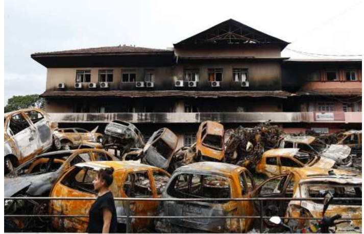
Nepal's Supreme Court left charred by fire from 9 September protest. The building has been declared unusable and the apex body has resumed limited operation in tented camps. Picture from Skanda Gautam.
